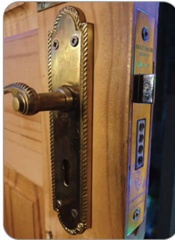
Figure 2-8: A mortise lockset installed in a door
